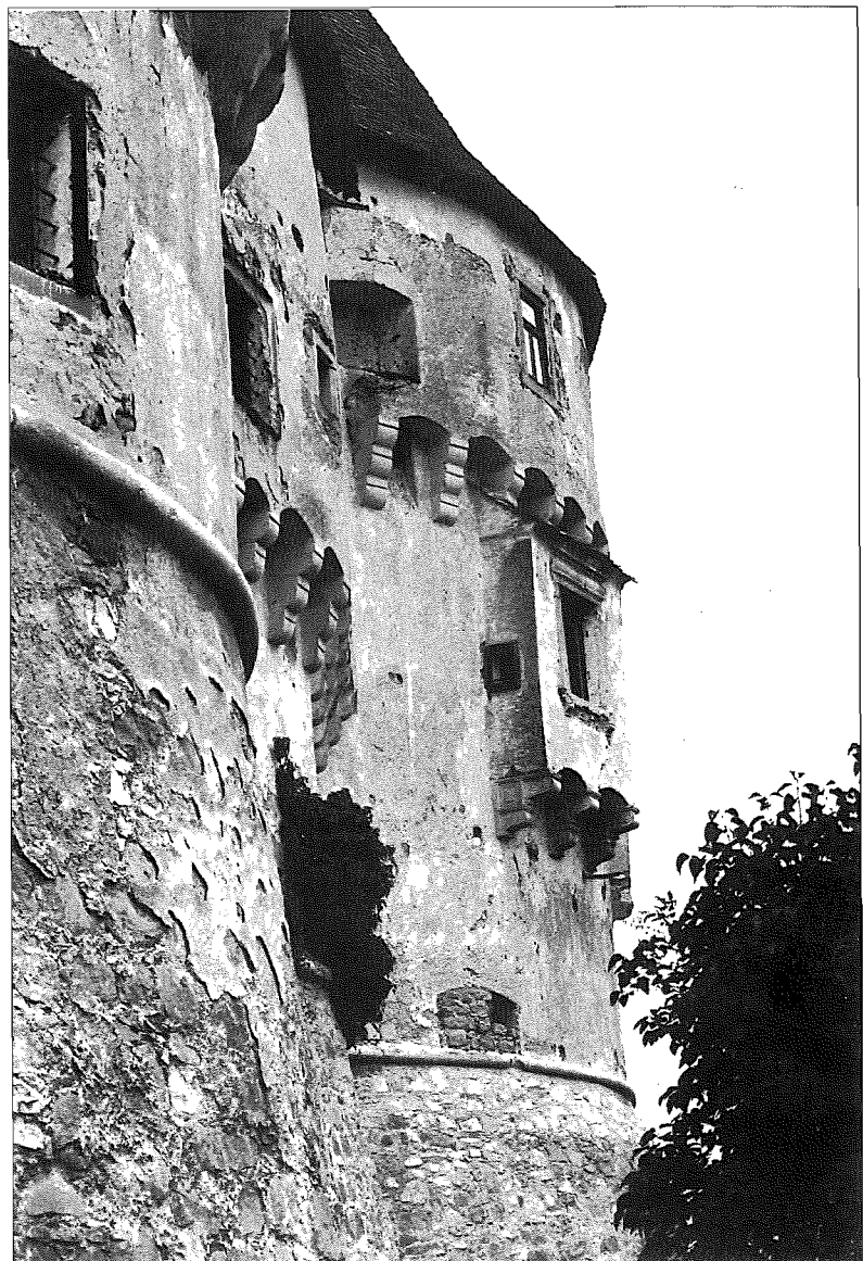
2 Zidovi dvorca Velikoga Tabora »izgrizeni« vlagom Walls of the castle of Veliki Tabor corroded by moisture.
